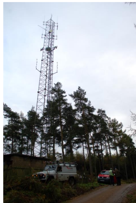
Utility radio tower hosting VHF Private Mobile Radio (PMR), UHF telemetry (SCADA) together with microwave fixed service backhaul.
