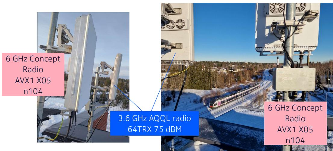
The field pilot demonstrated Nokia’s readiness to support the integration of the bandwidth of the new spectrum in the upper 6 GHz seamlessly into the mobile operators existing networks, allowing them to provide coverage from the existing macro cell sites.
